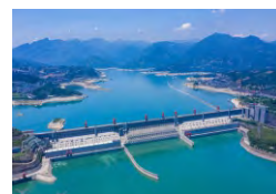
Power Station Reservoir
