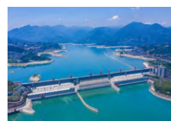
Power Station Reservoir
